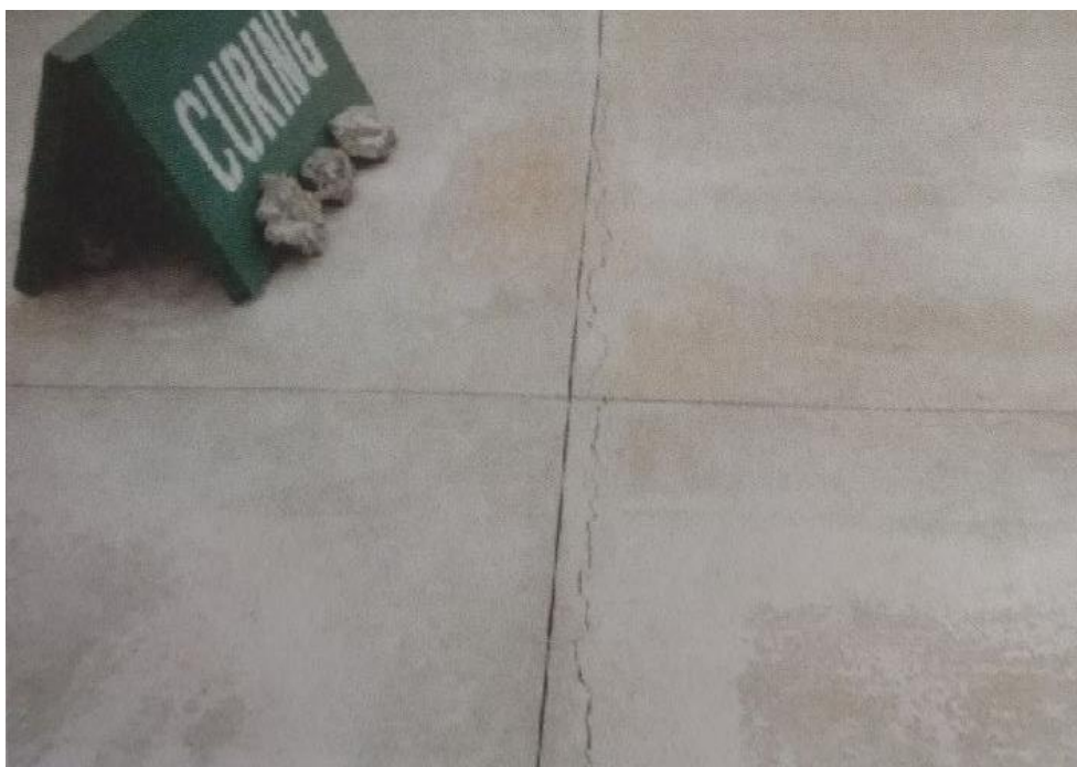
1- picture. Cracks in the seams.
